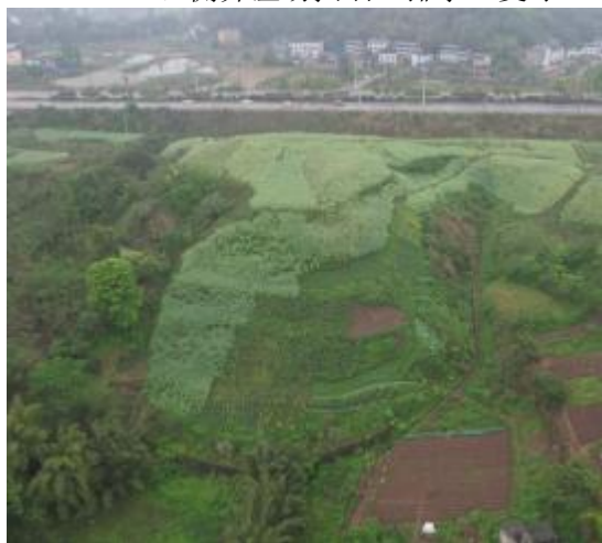
K39+300 左侧弃渣场挡墙、排水、复耕
